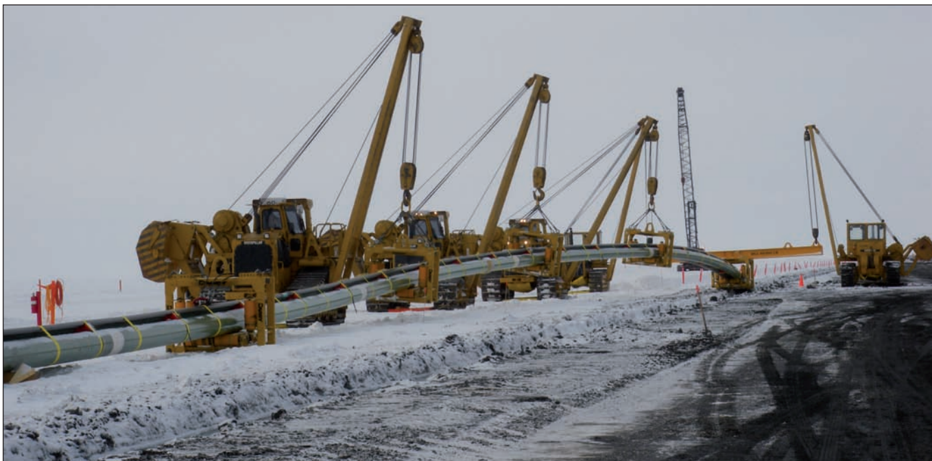
Sideboom pipelayers equipped with roller cradles are used to install the Nikaitchuq offshore flowline bundle through the ice slot into the subsea trench. The trench is cleaned out and surveyed prior to the equipment advancing to install another flowline bundle segment. INTECSEA joined the Nikaitchuq project in 2005, undertaking conceptual, pre-FEED and FEED prior to completing detailed design of the offshore flowline bundle in 2008 and providing onsite construction support during its installation the following year.
