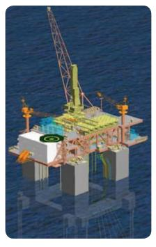
INTECSEA work over the years has played a significant part in helping Woodside conclude that the most appropriate deepwater development concept solution is a Tension Leg Platform with SCRs.
